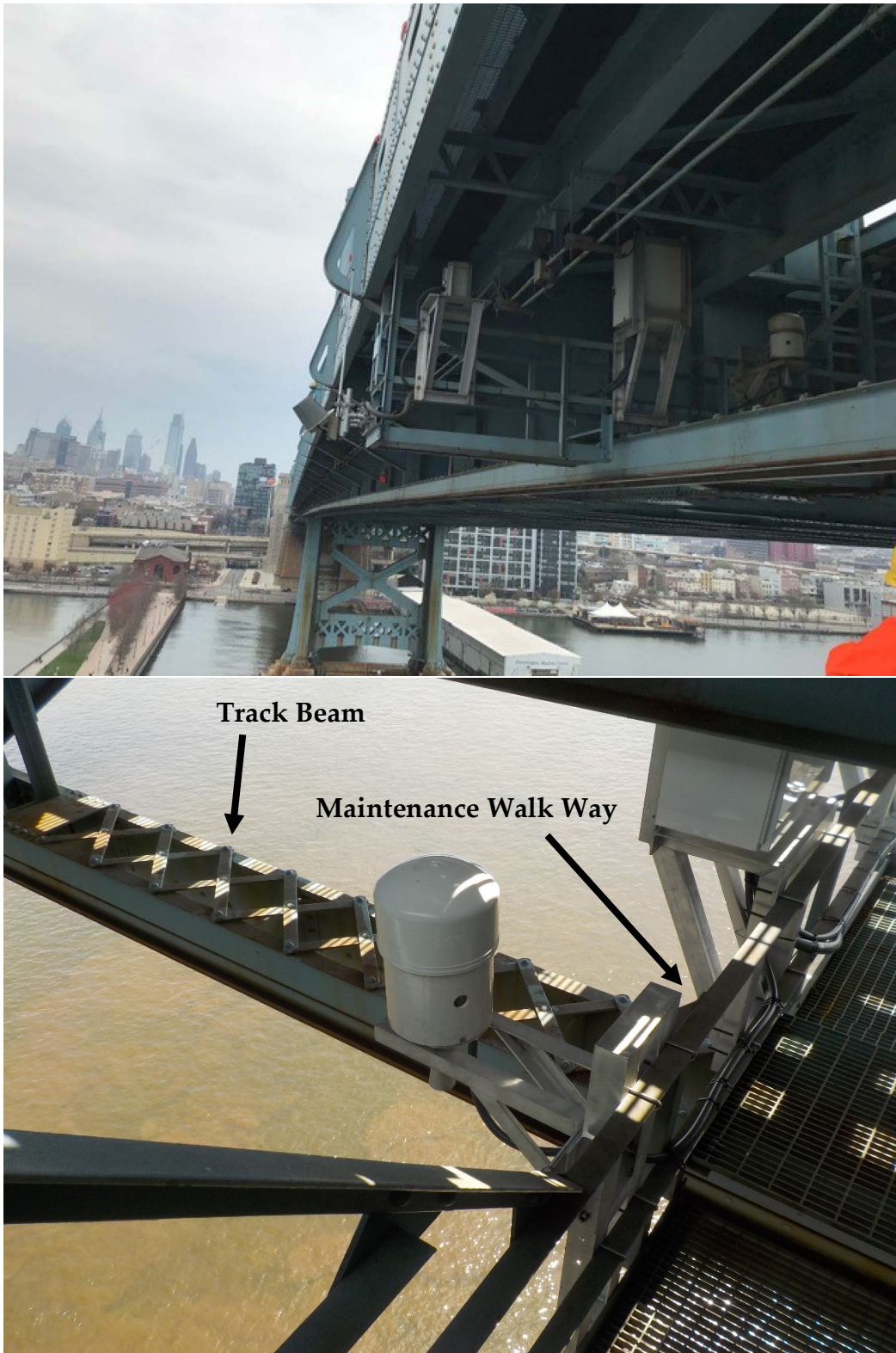
Images 1 and 2. Air Gap Sensor Installation on the Ben Franklin Bridge.
