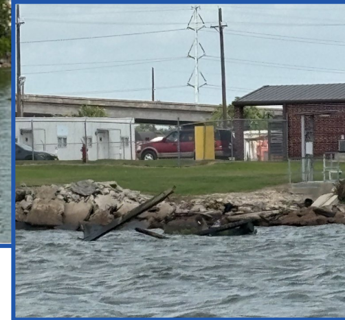
Port Arthur, TX
