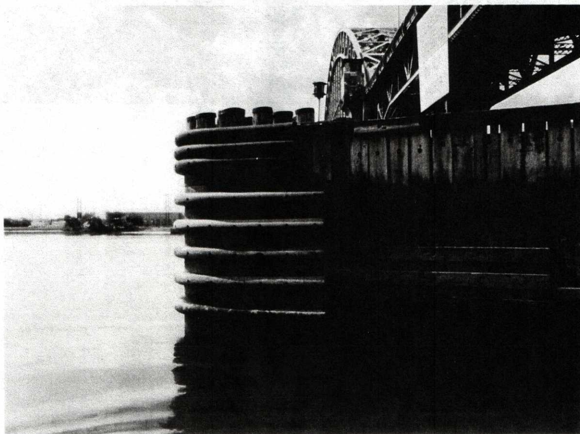
Downstream Fender of Pier F
